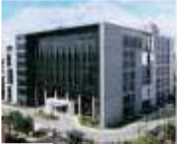
Taoyuan Technology Center (Green Building)
