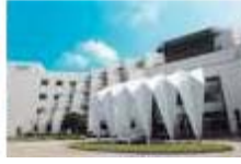
Tainan Plant (Diamond-rated Green Building)
